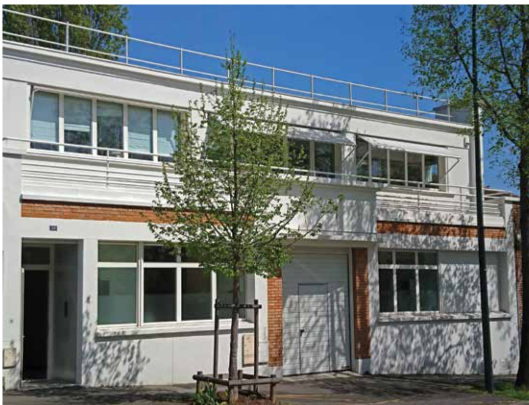
Neyco's Headquarter in Vanves, south of Paris (FRANCE).
