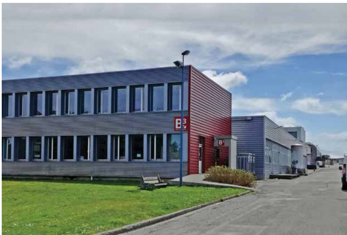
Our Plant in Lannion (FRANCE).
